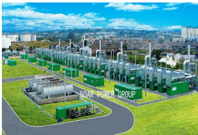
Containerized Power Plant (47MW: 9H21/32x28 Sets)
